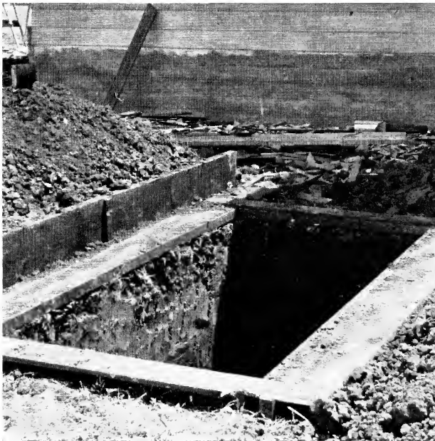
Fig. 5—Rectangular frame about the hole. The 2 × 10-inch planks are later used as baffle boards.
